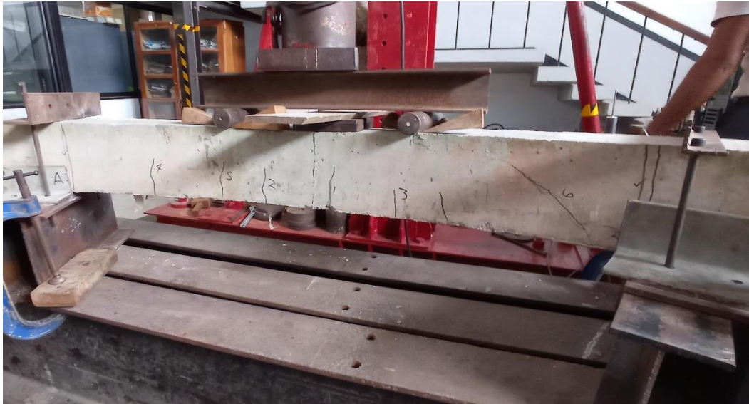
Figure 19: Cracks in a Beam 1-1-CO
