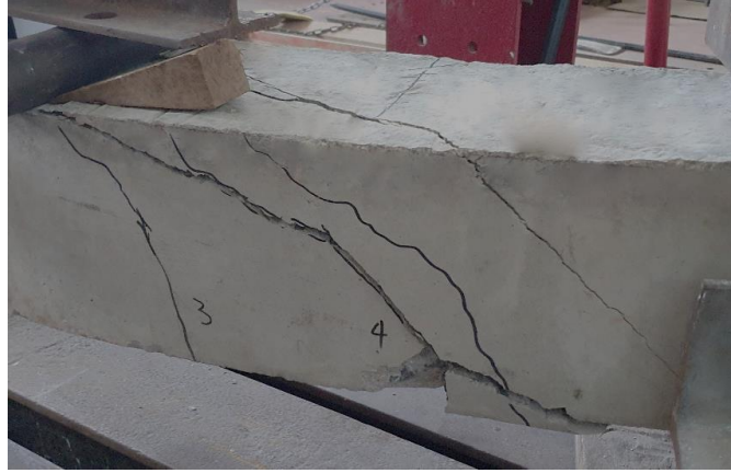
Figure 23: Shear + Torsional failure of Beam 1-2-CO
