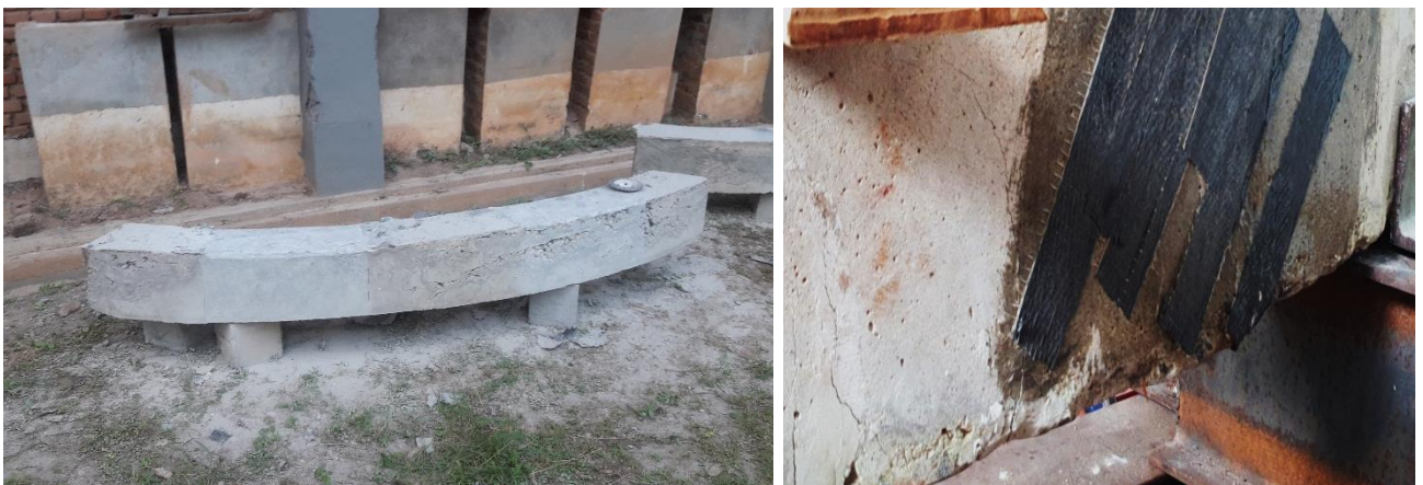
Figure 16: Surface preparation and CFRP fabric installation
