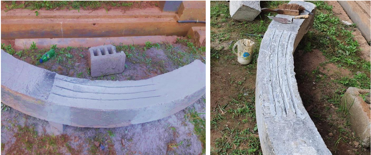
Figure 15: (a) Cutting grooves; (b) CFRP plate installation
