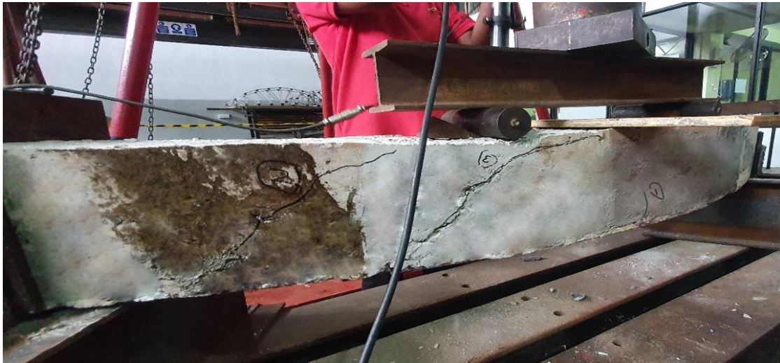
Figure 25: Cracks in a Beam 2-1-FS
