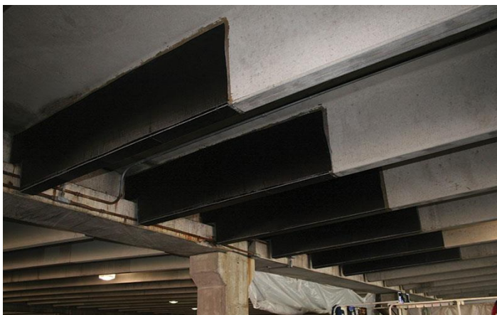
(a) wrapped over the webs of beams
