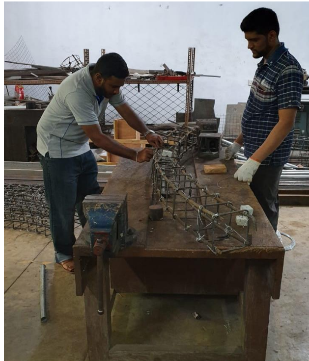
Figure 13: Steel formwork and reinforcement cage preparation
