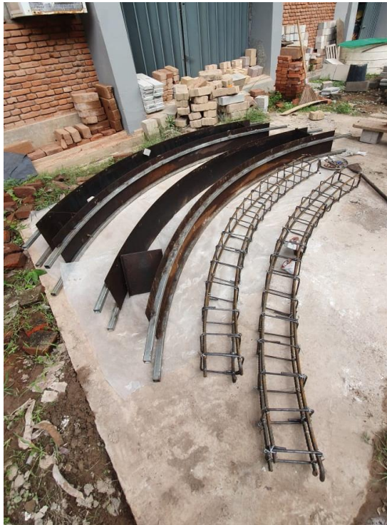
Figure 13: Steel formwork and reinforcement cage preparation
