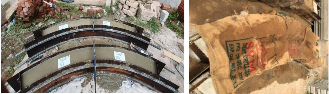
Figure 14: Beams cast and cured using gunny bags
