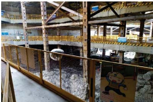
Temporary Supports at Site
