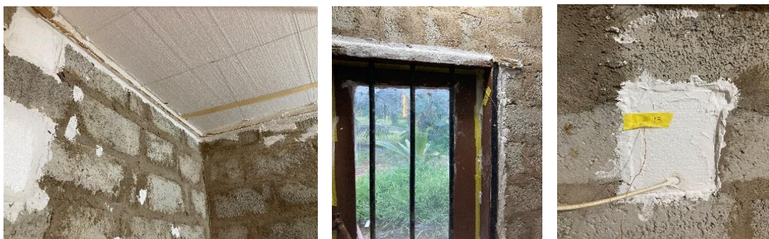
Figure 5-11: Preparing the interior for data collection – Air sealing the building interior
