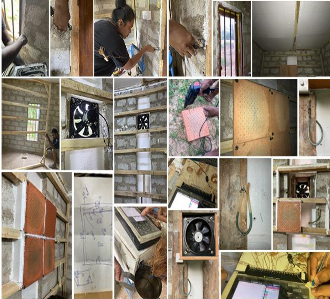
Figure 5-12: Preparation of the Prototype building for thermal investigation
