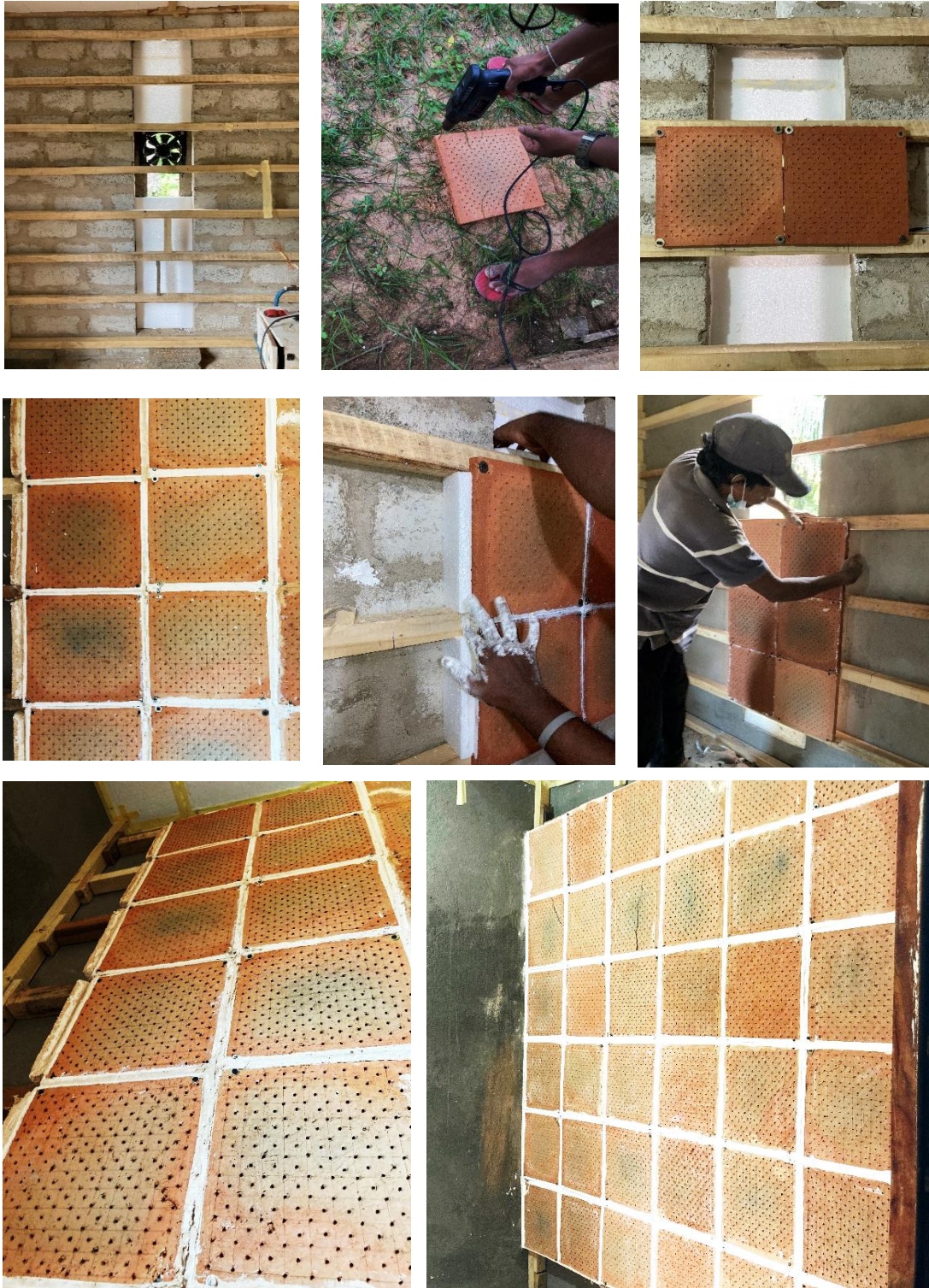
Figure 5-8: Installation of the DCDW panel; fixing the timber frame, drilling the panels, screwing, sealing, and finishing
