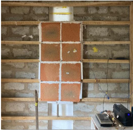
Figure 6-6: Application of the DCDW with 8- panels, 2- fans
