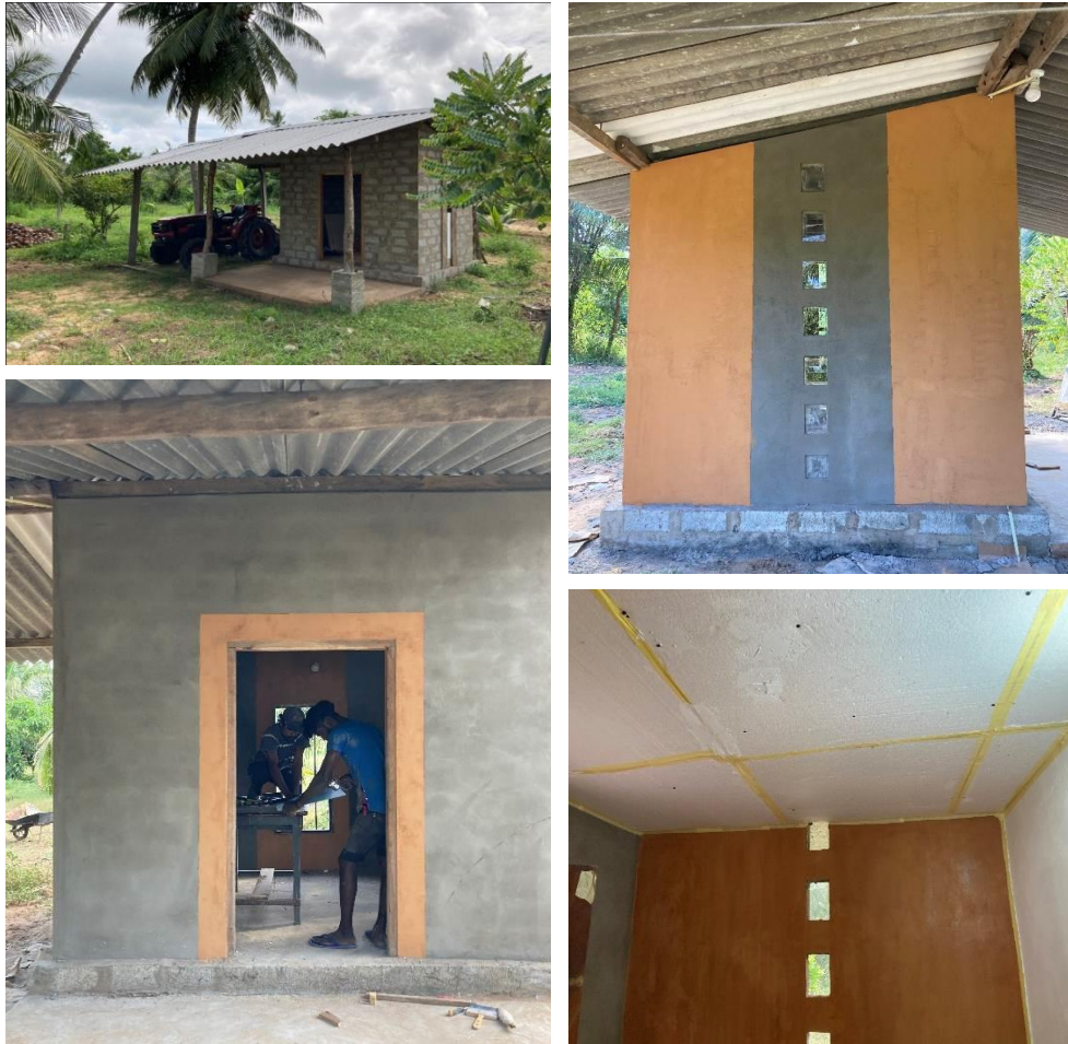
Figure 5-4: Outdoor and Indoor appearance of the real scale building with final finishes.
