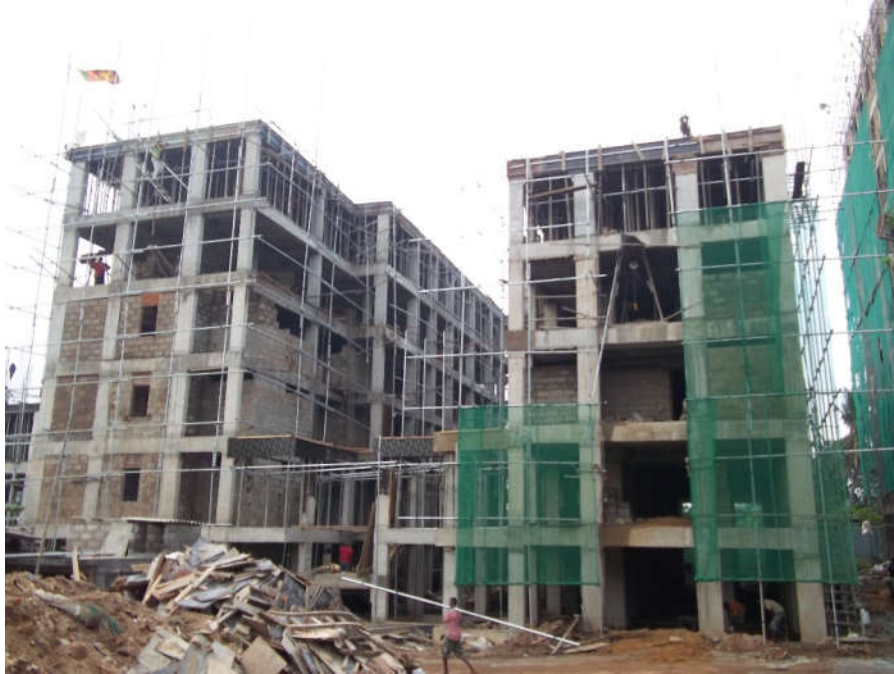
Figure 1:Formwork sorting at Angulana Site (State Engineering Corporation)
