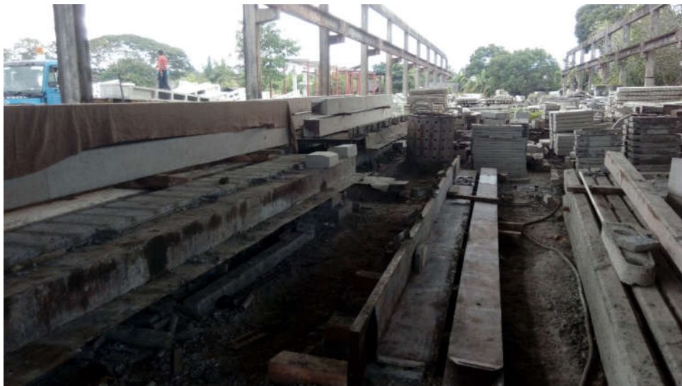
Figure 7:Precast concrete product from recyclables (SEC-Ekala)
