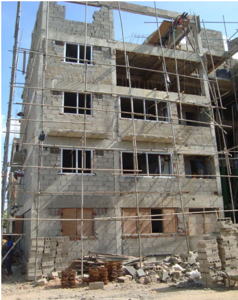
Figure 5: Inadequate site space for waste sorting and storing (Borella site-SEC)
