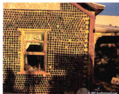
Fig 9. A house constructed with bear bottles as wall material
