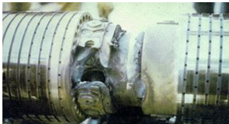
Fig. 1-2. Fracture of the shaft of generator at Mohave power station in 1970s [3].
