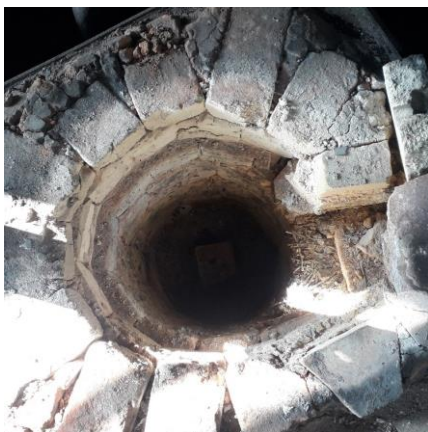
Figure 26-Improper construction of the pit furnace
