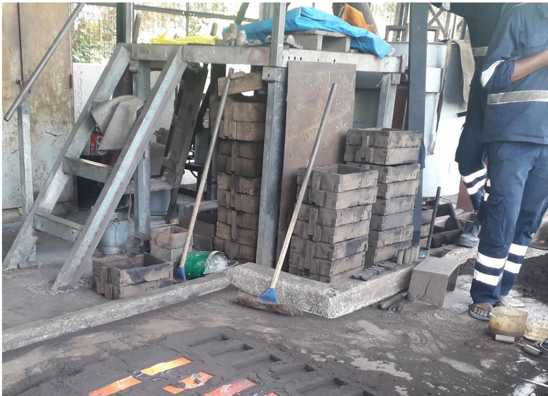
Figure 31: Tilting furnace covered with various materials due to non-use
