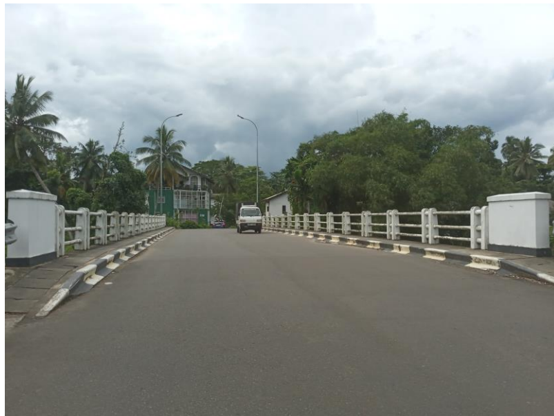
Figure 4.1. Bridge in Mudduwa Batugedara road in Rathnapura
