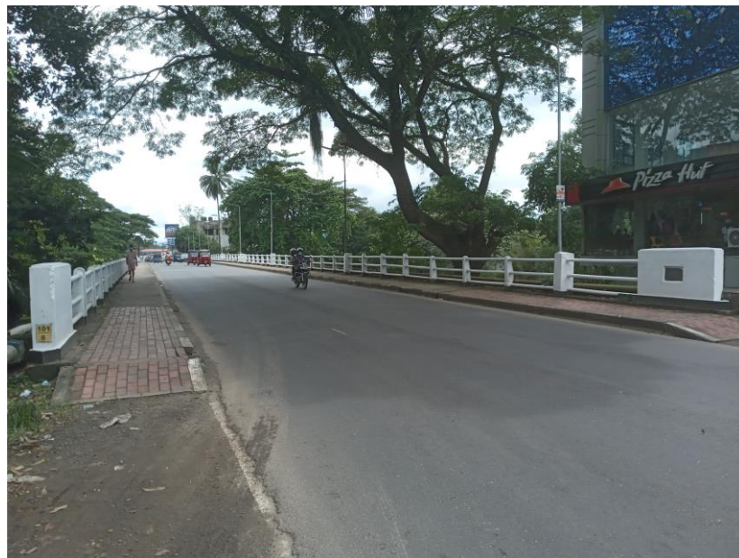
Figure 4.2. Bridge No. 101/6 Colombo-Rathnapura-Wellawaya road
