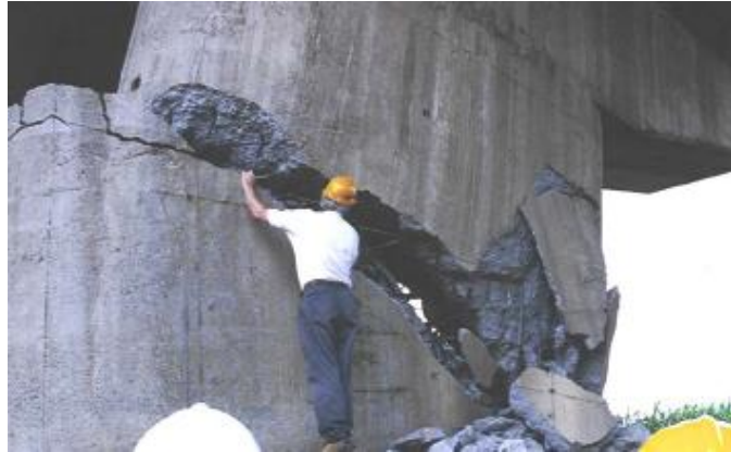
Figure 2.2. Substructure failure
