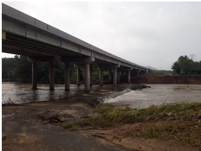
Figure 4.5. Mahaoya Bridge at 42+240 in Central Expressway
