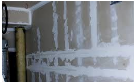
Figure 2.4– Application of Joint Compound
