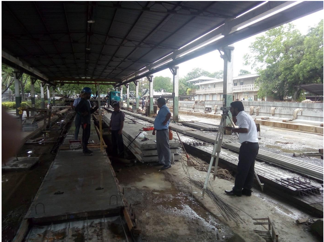
Figure 5.3.1 – Taking spot levels on prestressed panel before releasing the strands
