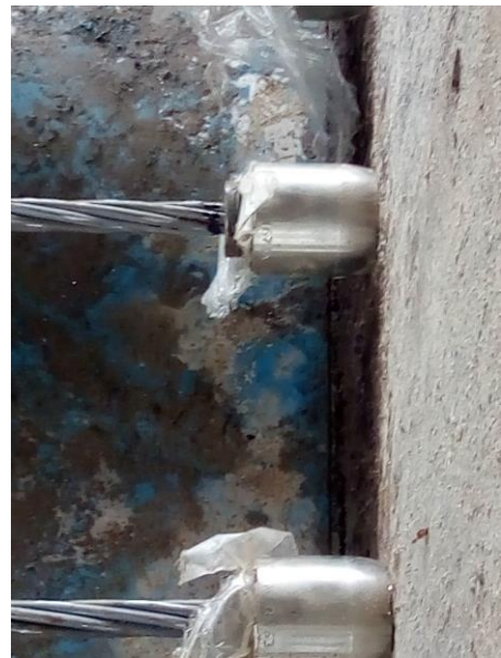
Figure 5.2.5 – Initial strand location marked at the jacking end
