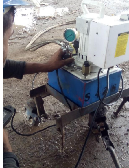
Figure 5.2.2 – Application of jacking force to strand.
