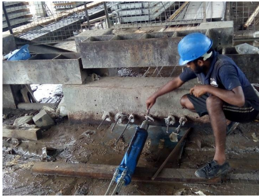
Figure 5.2.1 – Hydraulic jack connected to strand.
