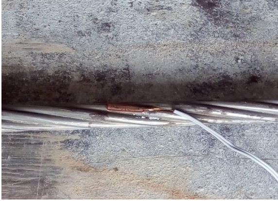
Figure 5.1.2 – Electronic strain gauge installed to strand
