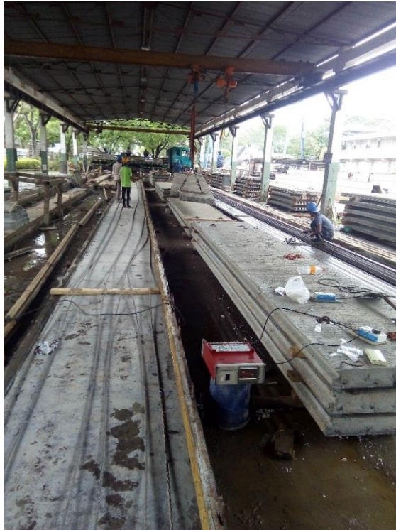
Figure 5.1.1 – Laying of strands on long line precast bed
