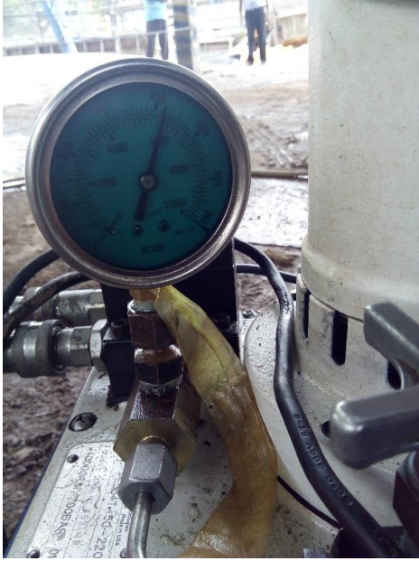
Figure 5.2.3 – Observation of applied jacking force from
