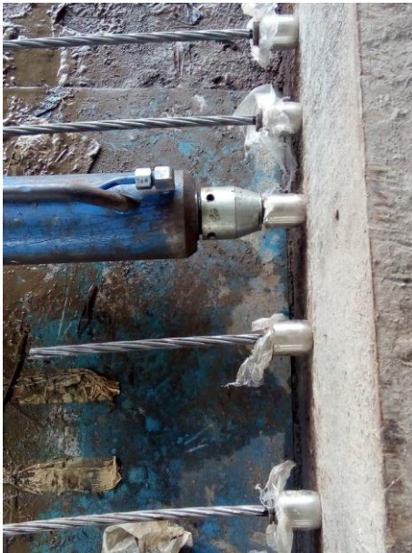
Figure 5.2.4 Hydraulic jack connected to strand
