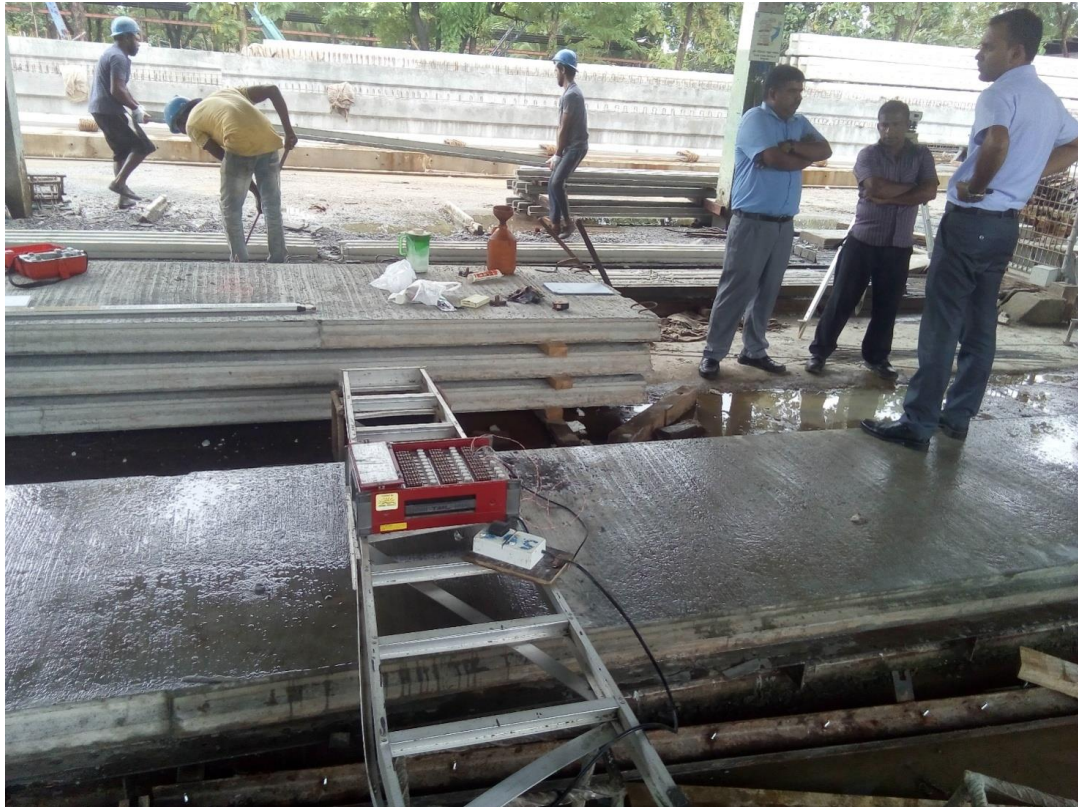
Figure 5.4.1 – Data logger set on a platform, not to disturb during strand releasing process
