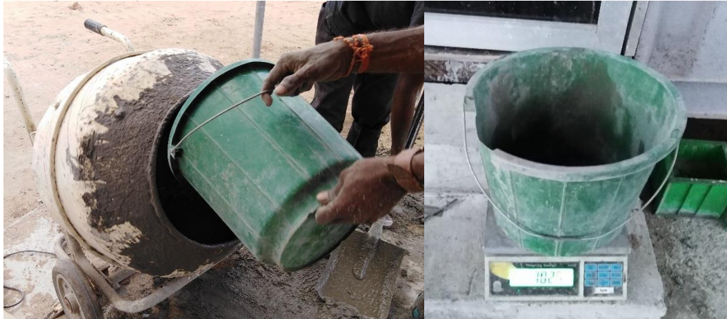
Figure 3-12 Mixing the concrete
