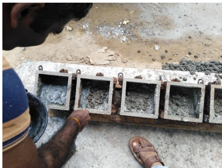
Figure 3-15 Applying the bonding agent
