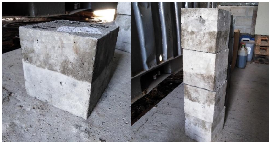
Figure 3-27 Cold joint with horizontal plane
