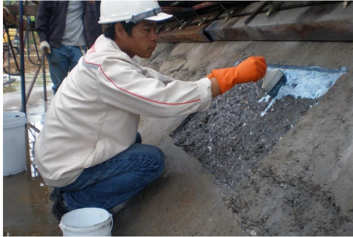
Figure 2-24 Application of bonding agent ( http://www.cormix.com/ )
