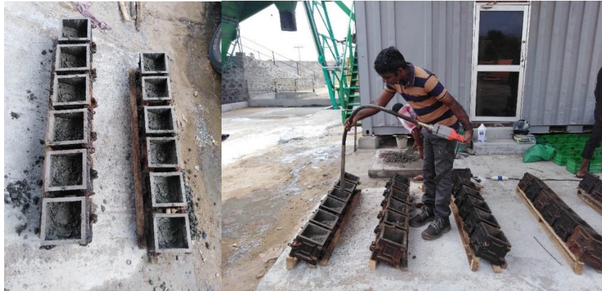
Figure 3-14 Casting and compacting the first layer of concrete
