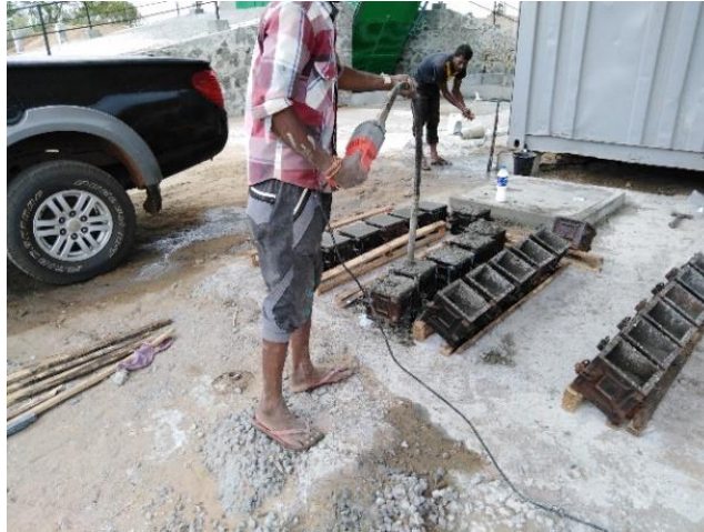
Figure 3-18 Casting and compacting of 2 nd layer for 1 hrs. delay
