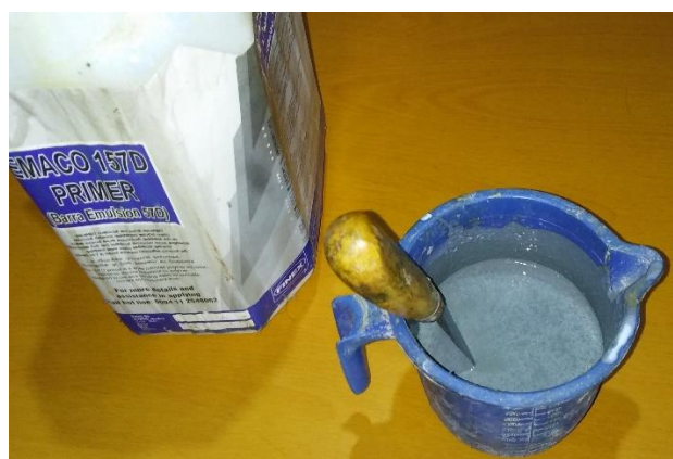
Figure 3-10 Preparation of bonding agent
