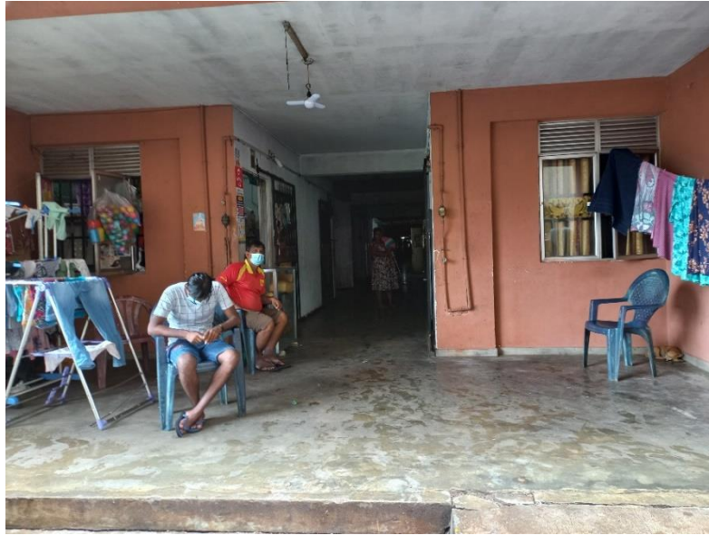
Image 4.20 – Internal Entrance Lobby of Block A in Muwaduru Uyana
