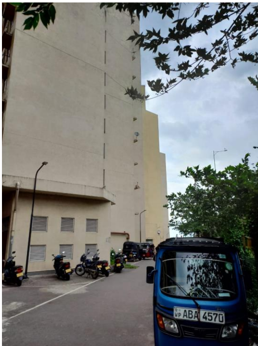
Image 4.35 – collective Blank façades in the side
