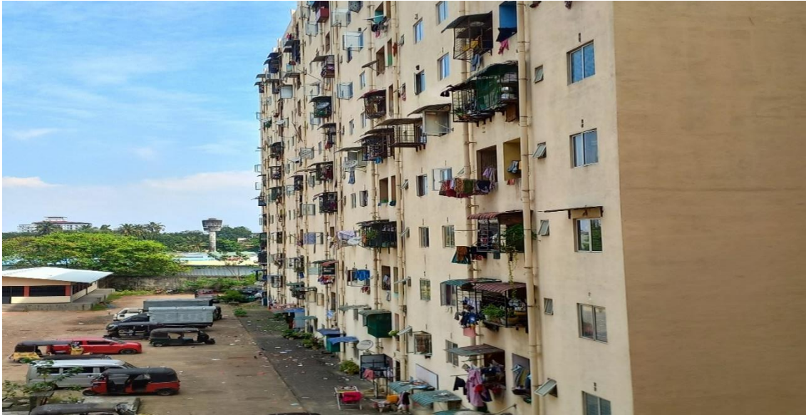
Image 4.69 – Long facade of Randiya Uyana
