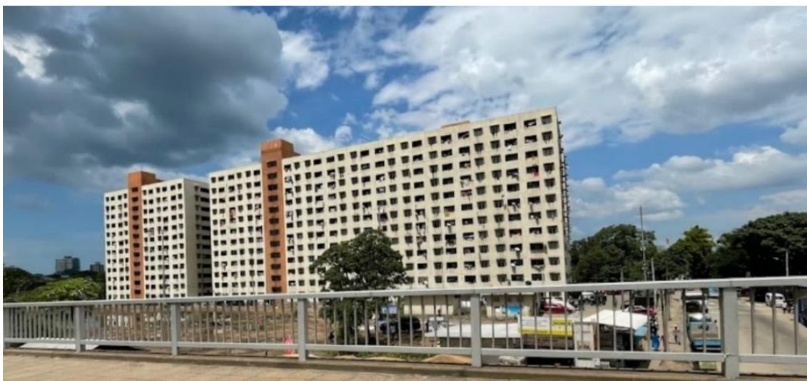
Image 4.2- View of Muwaduru Housing scheme from the bridge
