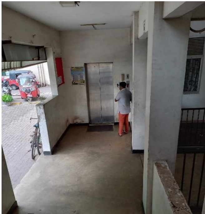
Image 4.65 – Lift opening to an open lobby immediately next to the access road
