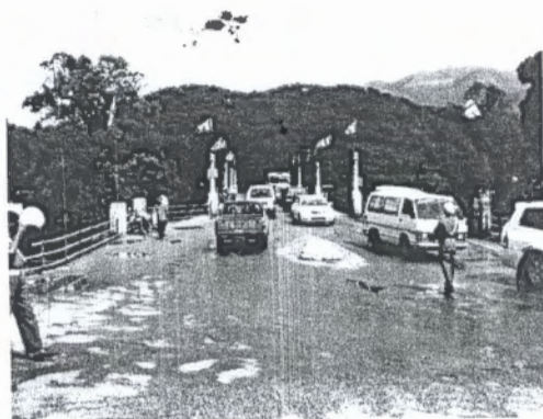
Fig.122: The bridge of Peradeniya as the beginning of the new approach
