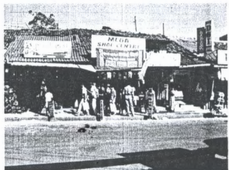
Fig 106: Low scale single storey shops creating the Final Transformation
