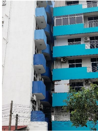
Figure 1.12: Lack of solar access in an 8-floor residential building in Dehiwela suburb
