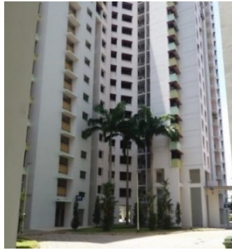
Figure 2.25: Overhangs, reveals, and balconies in a high-rise residential building in Singapore
