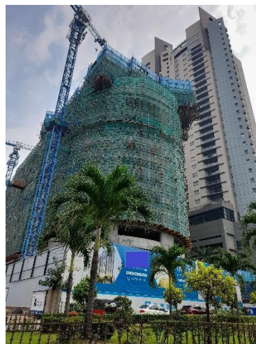
Figure 1.13: A new high-rise residential building of 40-floors being constructed close to an existing high-rise residential building affecting the view and solar access of the latter
