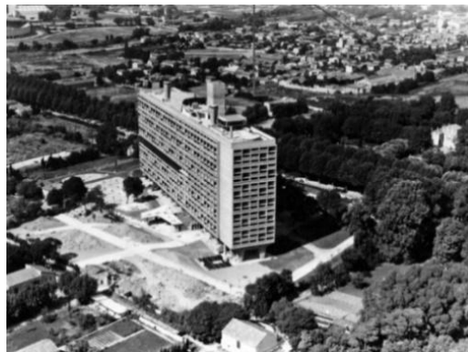
Figure 2.2: Unite de Habitation, Marseille by Le Corbusier
