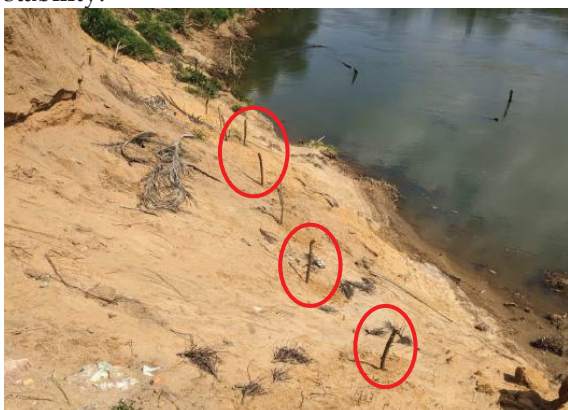
Figure 2 – Live poles of Hibiscus tiliaceus planted on a failed riverbank section
