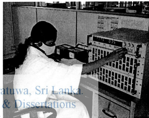
Figure 7.12: Electronic load connect to the battery discharging process
