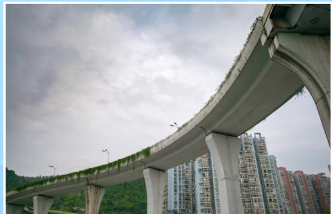
Fig. 2. A beam bridge carried on piers (overpass, Yunyan District) [5]. Image: lin2015, Pixabay, CC0.
