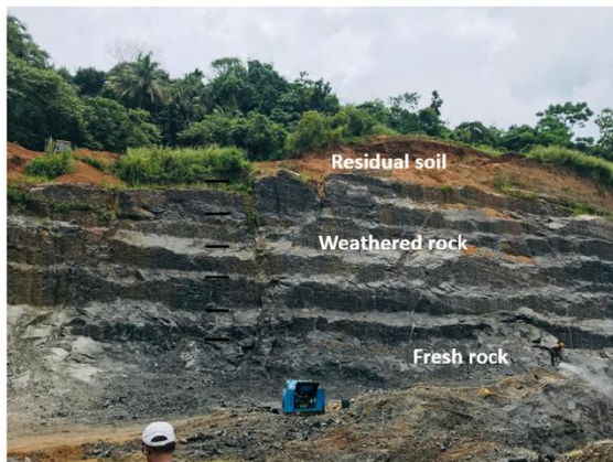
Figure 2: Location 1 - Granitic gneiss - ch. 6+155 km
