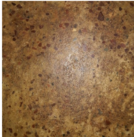
Figure 6-6: Appearance of final floor
