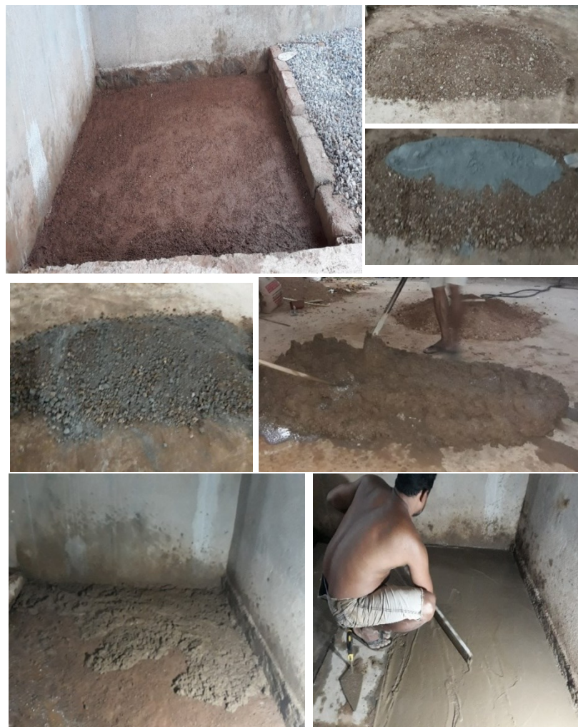
Figure 6-2: Floor construction work
