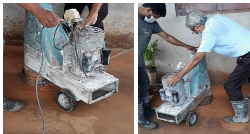
Figure 6-4: Floor surface cutting process with terrazzo machine
