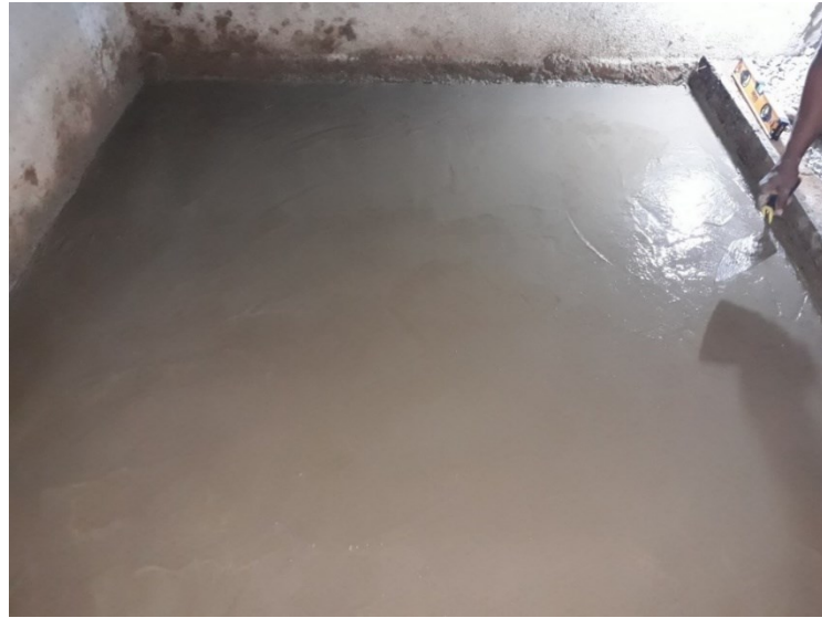
Figure 6-3: Soil concrete floor in the green state
