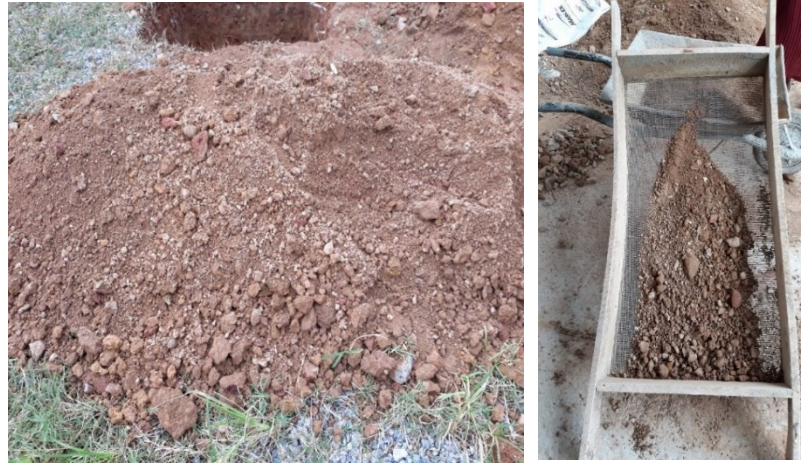
Figure 6-1: Extracted soil for floor construction and the soil sieving process to remove larger particles
