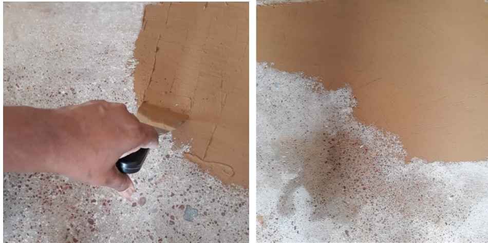
Figure 6-5: Clay slurry application
