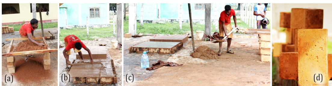
Fig. 6.32 Manufacturing mud concrete block
