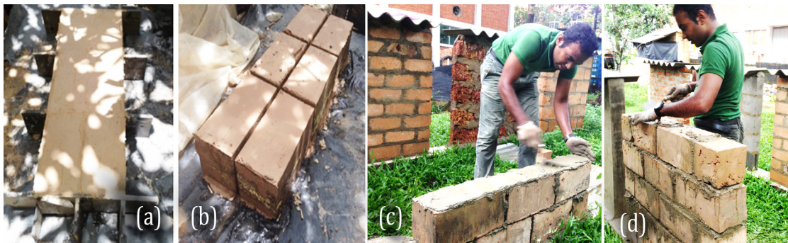
Fig. 5.9 Construction of geopolymer wall sample
