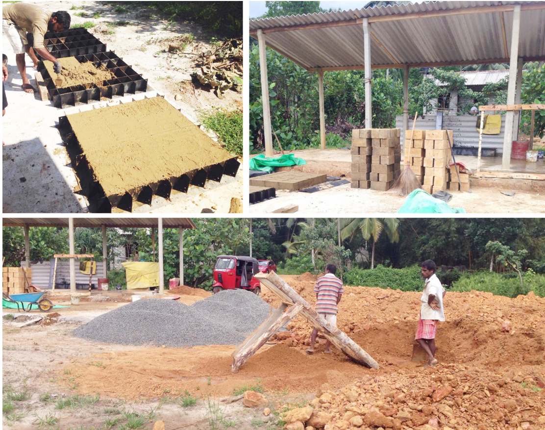
Fig. 6.35 Technology transferring to villagers to build their houses
