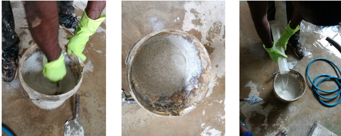
Fig. 3.3 Adding activators additives to mud concrete block mix
