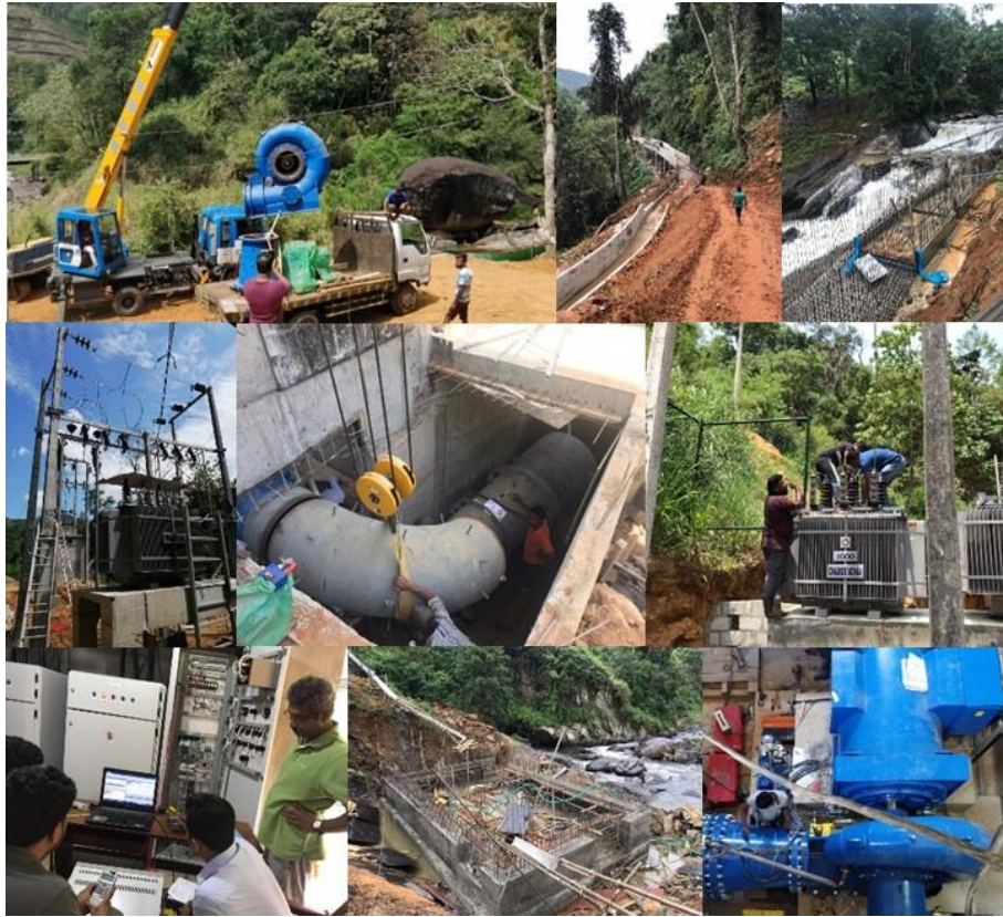
Figure 2: Construction of mini hydro power plant in Sri Lanka (Hulu Ganga mini hydro power plant)
