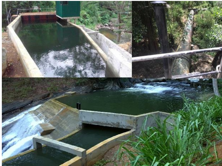
Figure 4: weir, intake canal, forebay and penstock of “Moragaha Oya” mini hydro power plant
