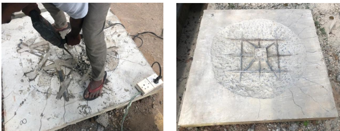
Figure 3. 4. Demolishing Concrete in the Cracked Area
