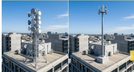
Different types of towers installed
