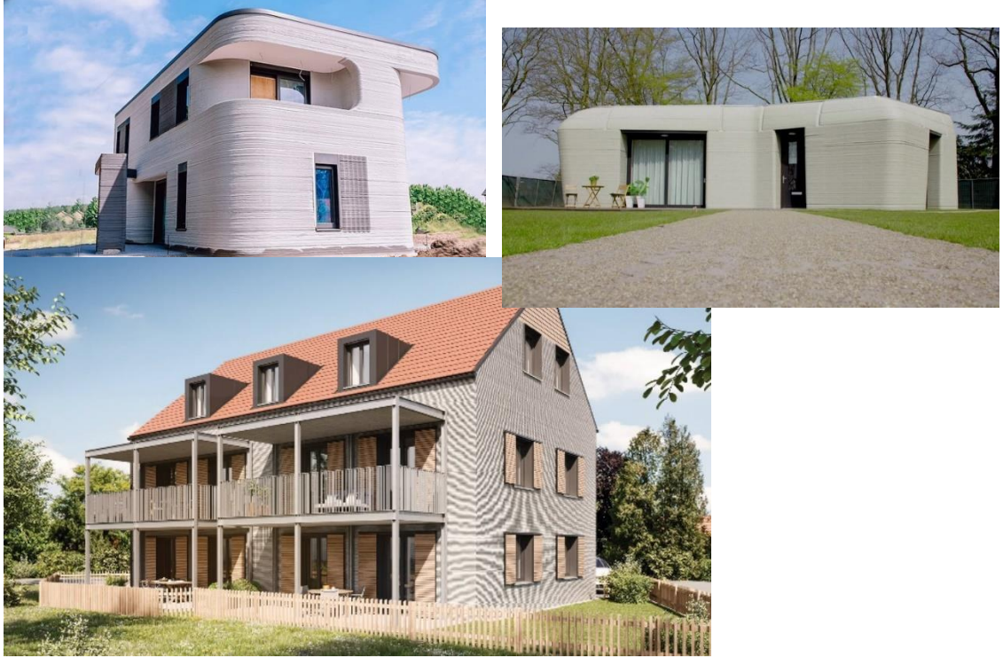
Figure 4.5: Plastering is not required for 3D printed houses (Ozdemir, 2021) (STIRWorld, 2020) (ABC Wires, 2021)
