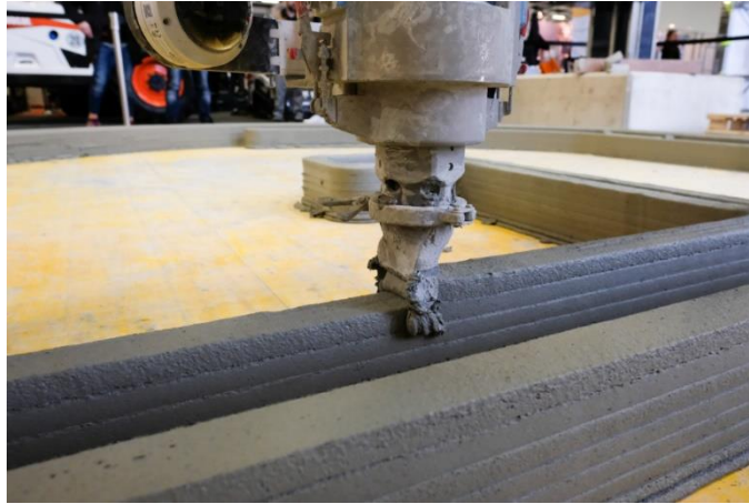
Figure 2.10: Print head of a gantry type printer
