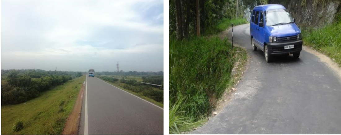
Figure 5.8. Roadside vertical drops and steep roadside slopes
