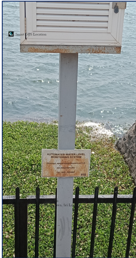
Figure 3-14: Automated water level monitoring system at Nachchaduwa Reservoir
