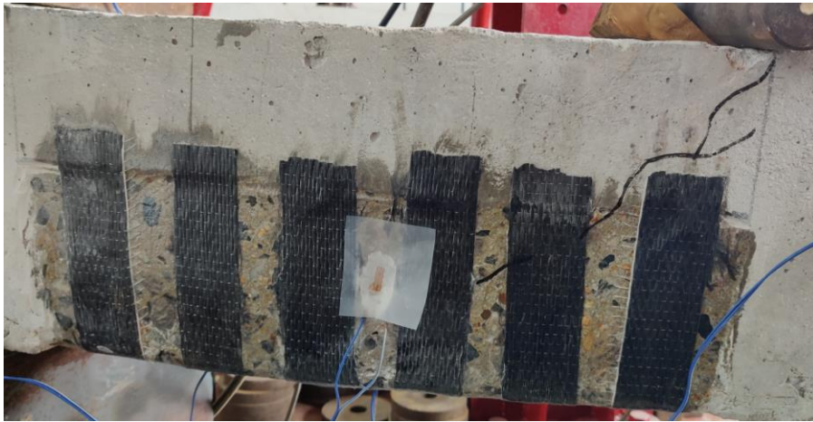
Figure 52: Cracks propagating with an inclination
