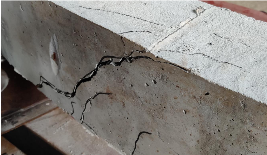
Figure 45: Shear failure of a control beam
