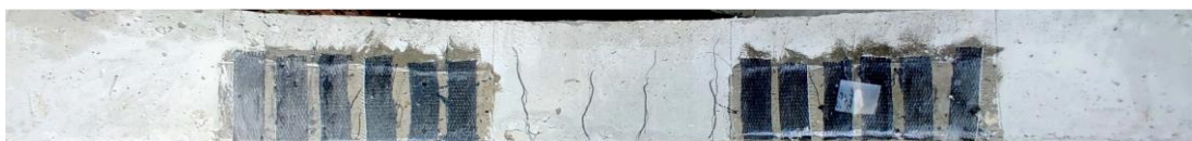
Figure 48: Initial flexural cracks
