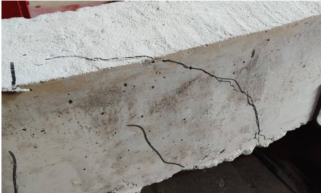
Figure 47: Shear failure of a control beam
