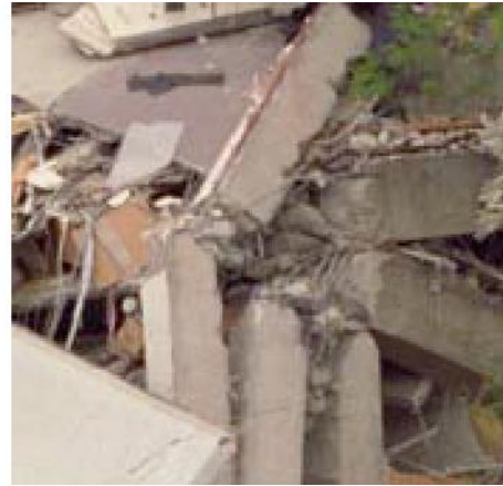
Figure 7: Failure modes of columns (a) Compressive failure of concrete and steel (b) buckling (Arya, 2009).
