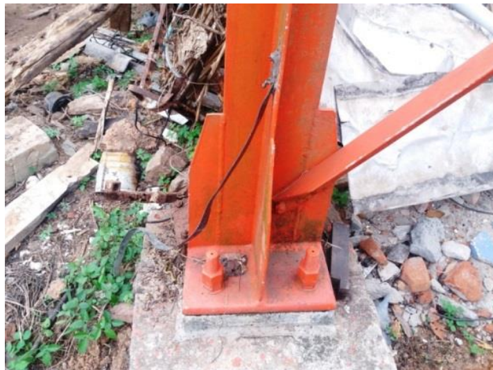
Fig. 1.3- Typical tower baseplate
