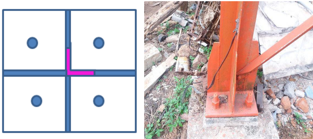
Fig 4.1- Typical baseplate of a lattice tower
