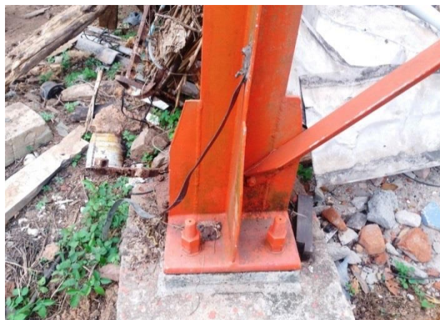
b) Baseplate with anchor bolts (SLT tower at Dambulla)
