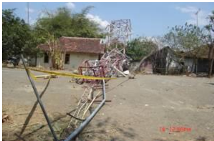
Fig. 1.2 – A tower reported to be collapsed in Pandang earthquake 2009, Indonesia (Razak, 2015)
