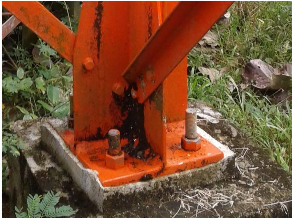
Fig. 5.1 -Typical view of a tower baseplate
