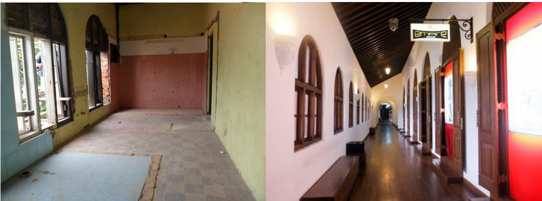
Figure 45 Before and after renovations
