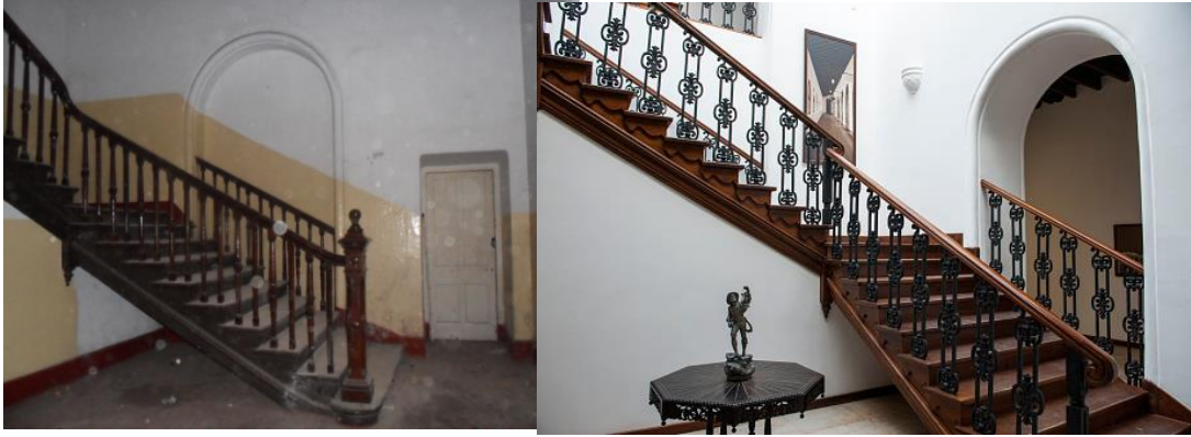
Figure 44 Before and After Renovations
