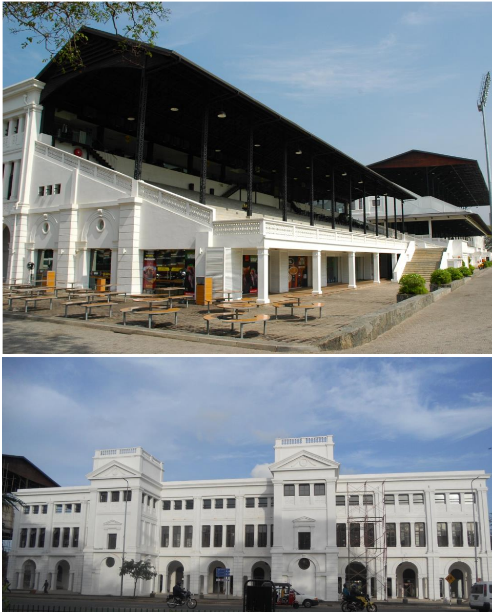
Figure 34 New Racecourse building
