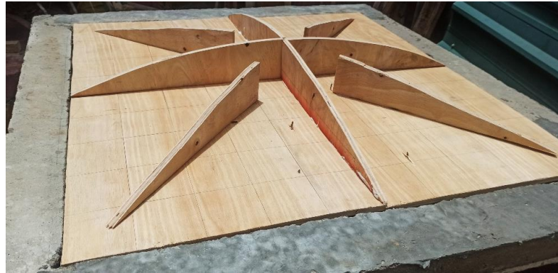
Figure 3-22: Arch shaped segments fixed to the formwork to get the desired shape
