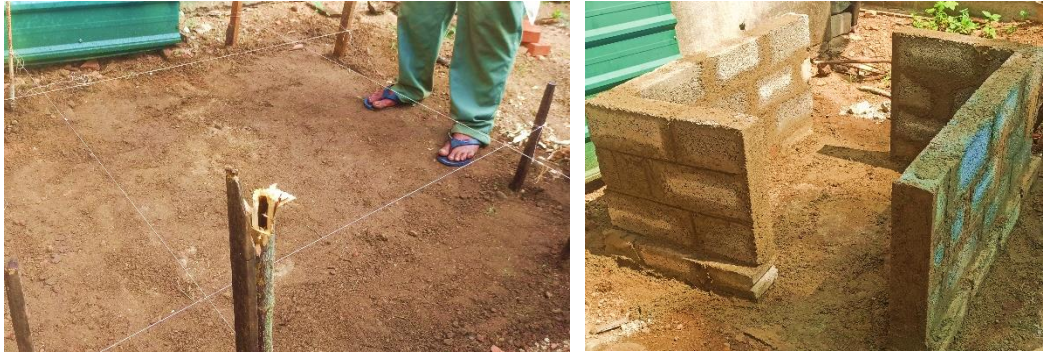
Figure 3-20: Setting out & construction of wall segments
