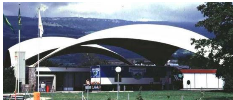
Figure 2-19: Highway service area Deitingen south, triangle concrete cupola roofs, Switzerland, 1968- Heinz Isler Source: (Chilton and Chuang, 2017)
