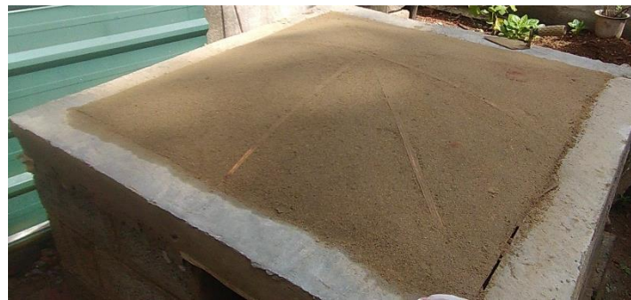
Figure 3-23: Finished surface with cement mortar
