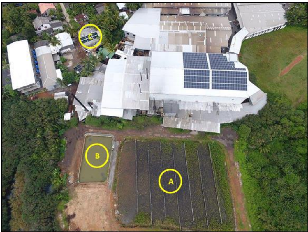
Figure 5-1: Photographic observations of the constructed wetland and the fishpond. A: Constructed wetland, B: Fishpond, C: Existing WWTP
