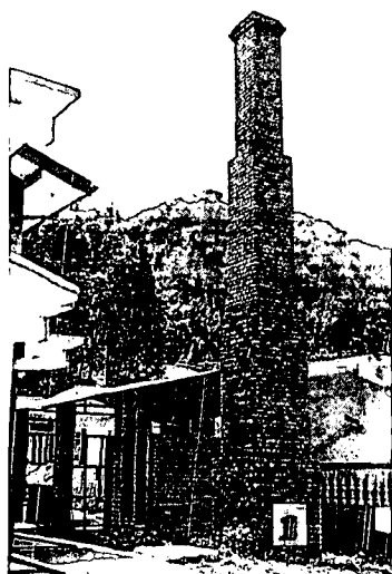
Figure 3.18 Abandoned incinerator in the Nuwara-Eliya hospital
