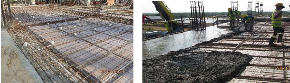
Figure 4.11: Preparation for topping concrete and Topping concrete pouring
