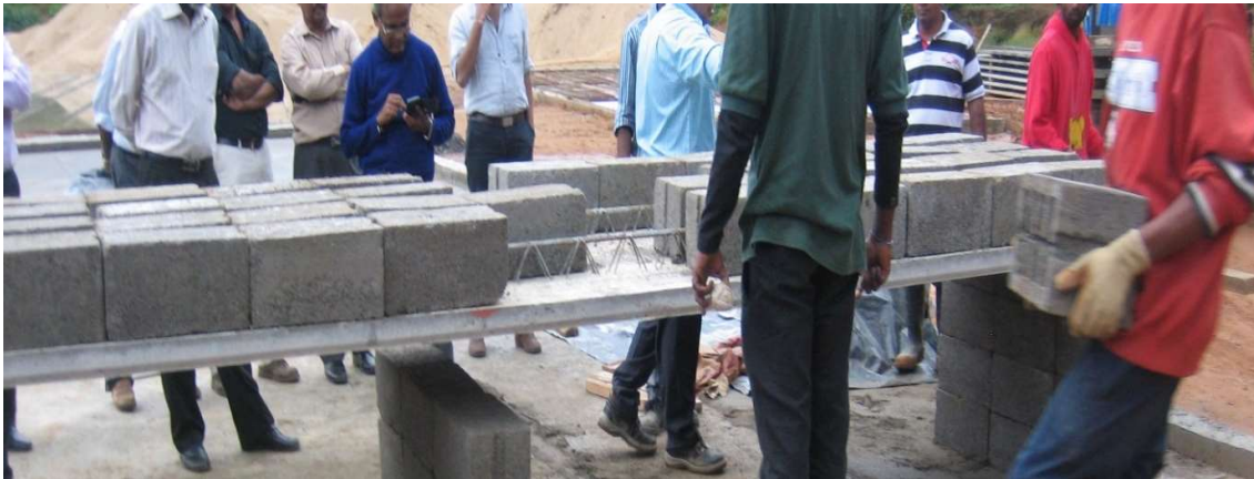
Figure 4.14: Load testing for Precast Palnk Salb panel at site
