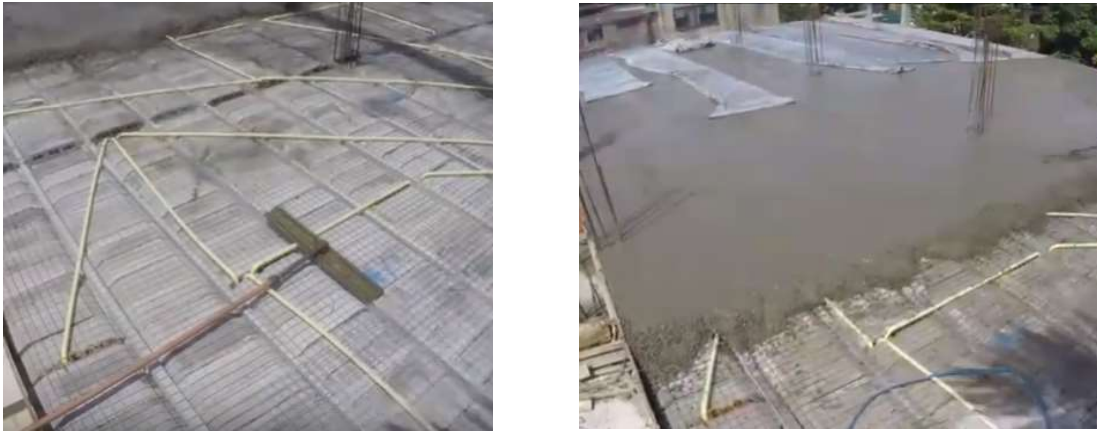
Figure 4.23: Arrangement for Topping concrete and pouring of 50mm thick concrete layer
