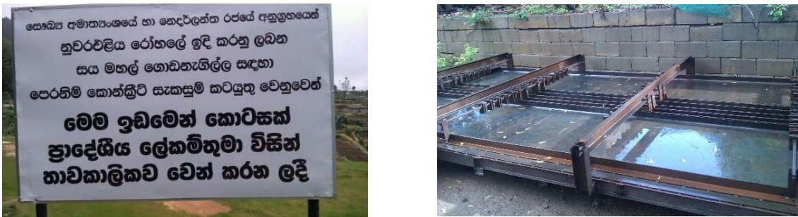
Figure 4.6: Ground Reservation for panel casting and Mold used in Nuwara Eliya project within the tanks
