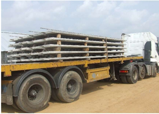
Figure 4.7: Slab Panel Transport arrangement and Slab Panel Stacking System
