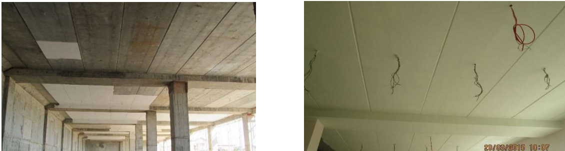
Figure 4.12: Bottom surface appearance and finished slab soffit
