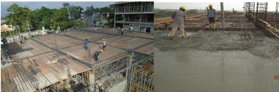
Figure 4.19: Reinforcement for conventional slab and Concrete pouring using pump car
