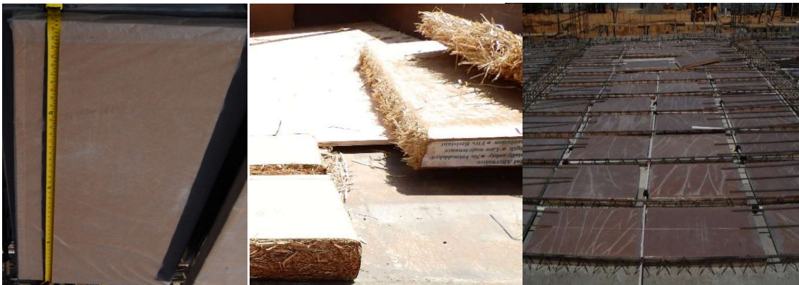
Figure 4.10: Straw Boards and Straw board laying on Precast Slab
