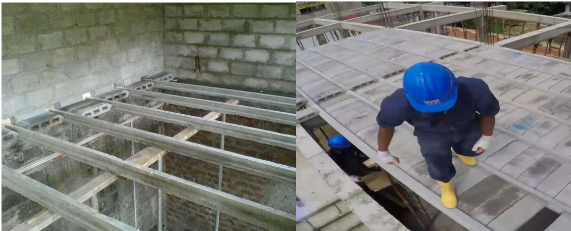
Figure 4.22: T-Beam Installation at site and Cement Block Installation at site
