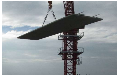
Figure 4.8: Slab Panel Hanging Device and Slab Panel Lifting by tower crane
