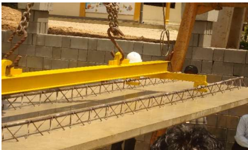
Figure 4.8: Slab Panel Hanging Device and Slab Panel Lifting by tower crane
