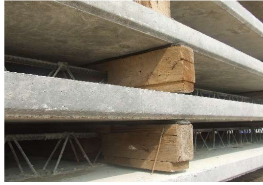
Figure 4.7: Slab Panel Transport arrangement and Slab Panel Stacking System
